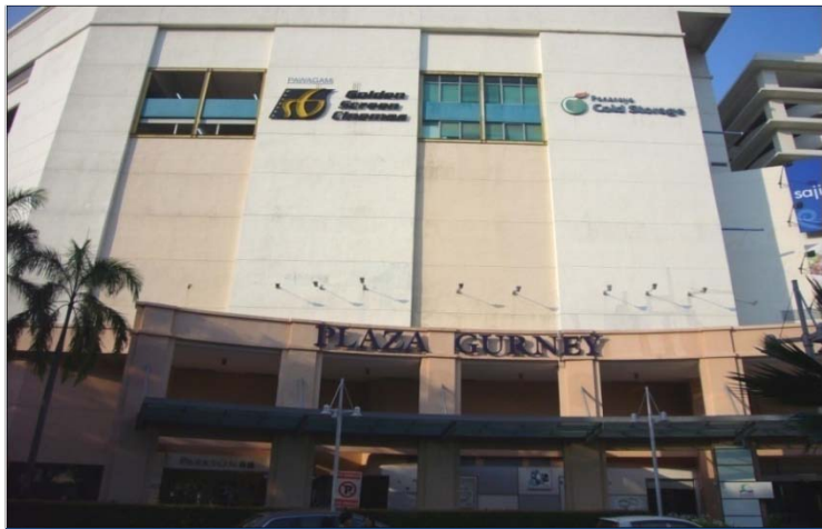
Before repainting of building facade
