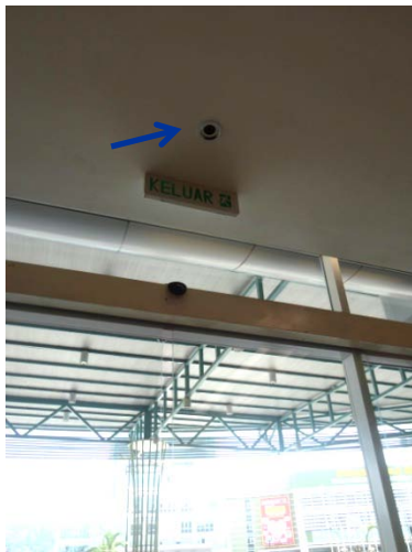
Installation of shopper traffic counters
