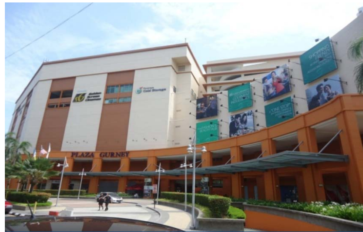
After repainting of building facade
