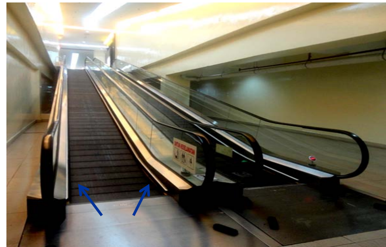
Installation of skirt brushes for travellers
