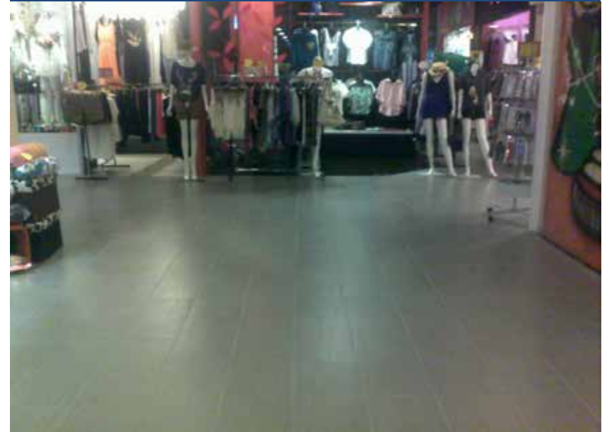
After - New Tiles
